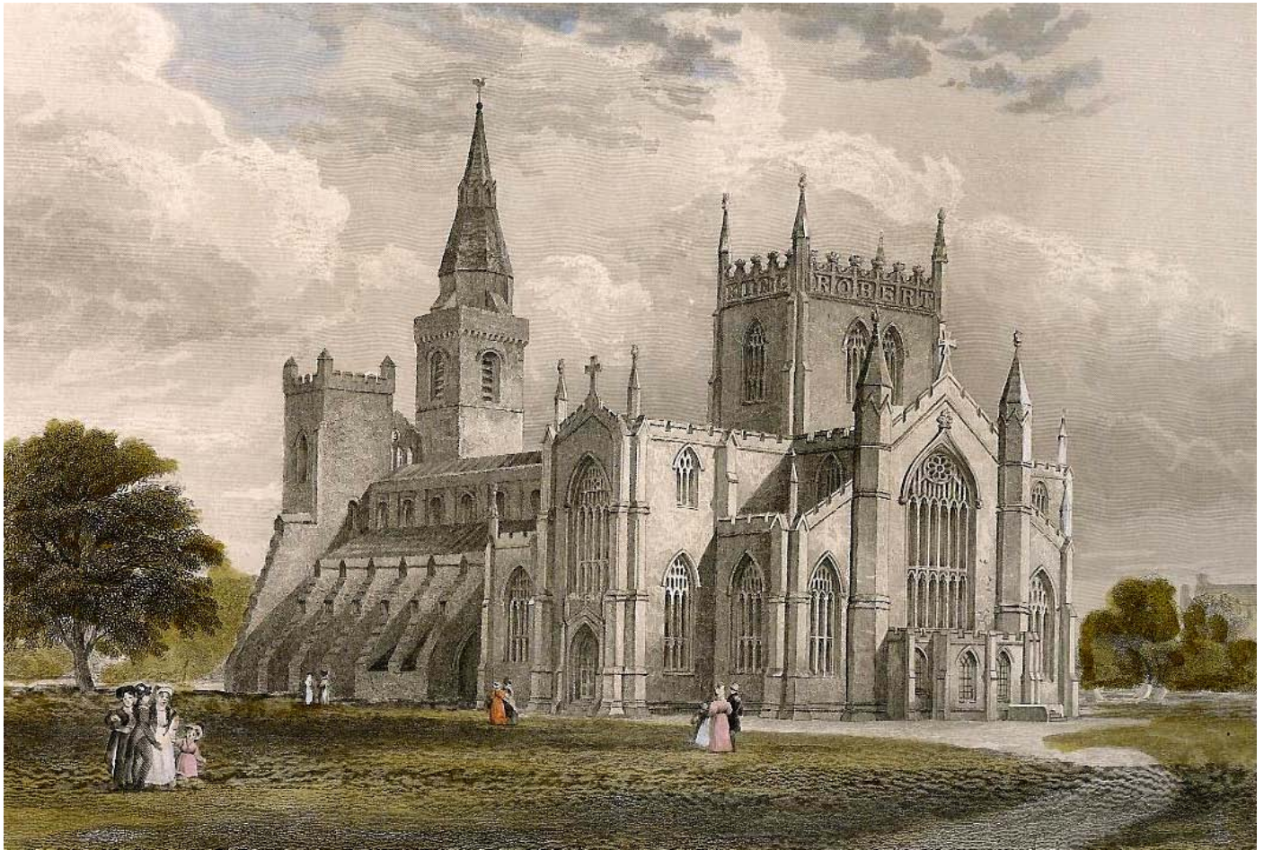
The Nave with the -New Abbey Church dedicated 1821.
