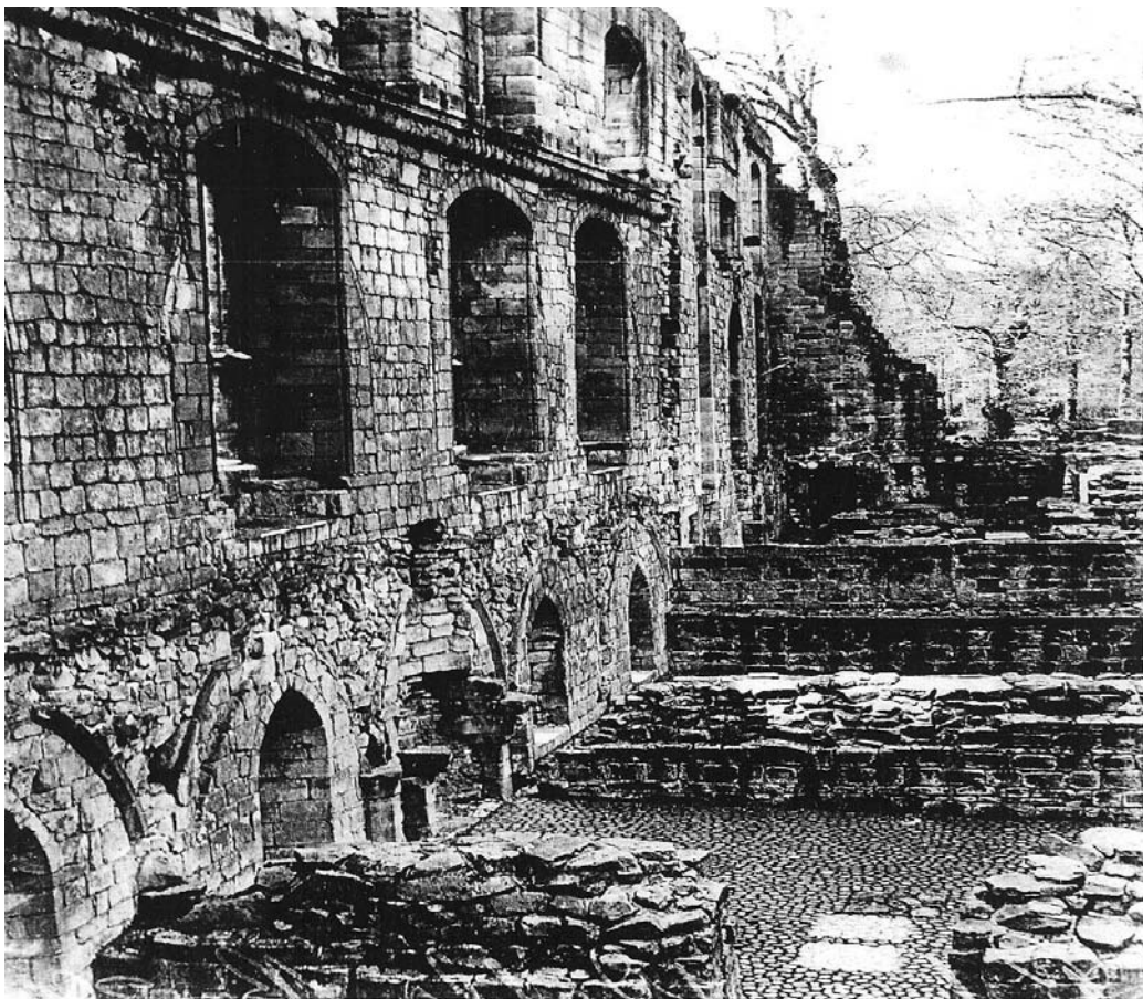
Palace north side.
